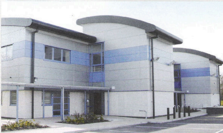
Completed third phase of CBTC
